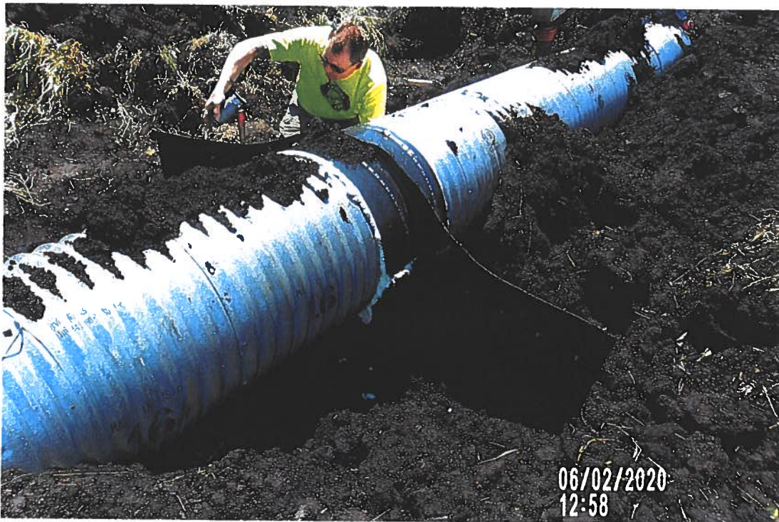
PICTURE # 3637 IS LOOKING SE SHOWING CREW USING FOAM FILL TO SEAL BETWEEN HDPE ANTISEEP COLLAR AND 24" CMP SURFACE DRAIN. (SUDAS SHOWS SHOULD BE BITUMINOUS MATERIAL)
