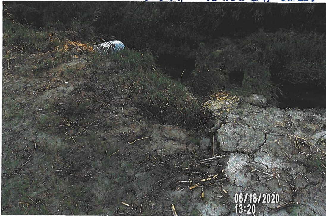
PICTURE# 3832 IS LOOKING SE SHOWING DD NORTH BANK NEEDING DRESSED UP ON WEST SIDE OF NEW CMP OUTLET
