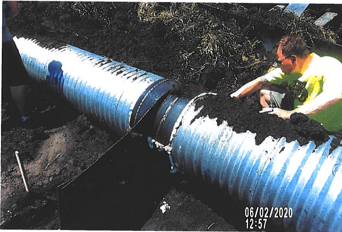
PICTURE # 3636 IS LOOKING EAST SHOWING CREW USING FOAM FILL TO SEAL BETWEEN HDPE ANTISEEP COLLAR AND 24" CMP SURFACE DRAIN, (SUDAS SHOWS SHOULD BE BITUMINOUS MATERIAL)
