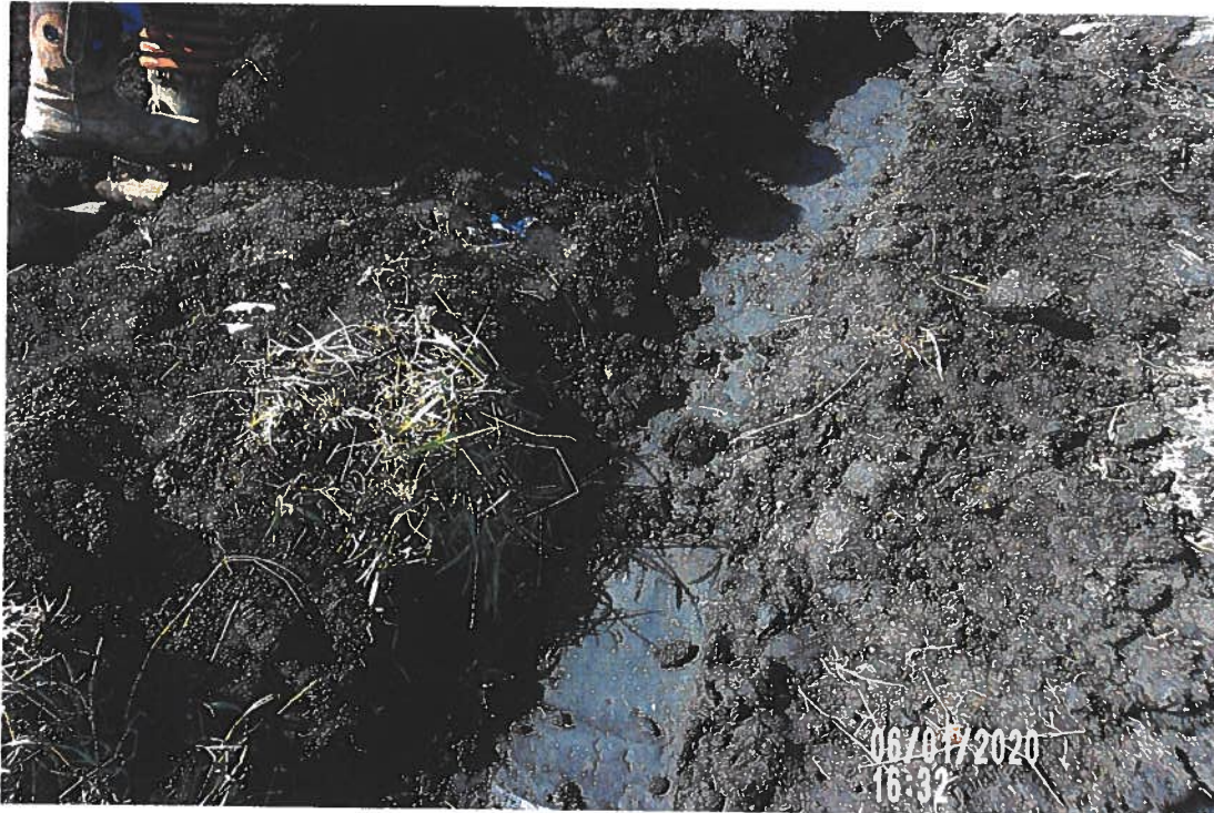
PICTURE # 3626 IS LOOKING SOUTH SHOWING SOIL COMPACTED ON SIDE OF NBW 24" CMP
