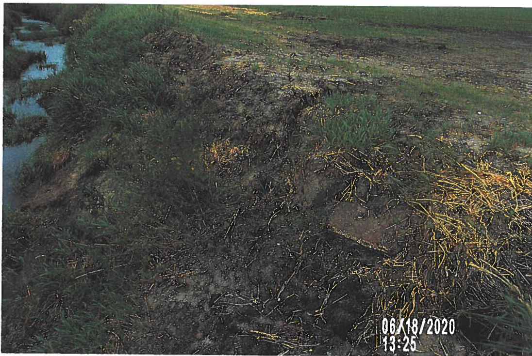
PICTURE # 3840 IS LOOKING NW OF NEW 24" SURFACE DRAIN SHOWING NORTH BANK WEEDING DRESSED UP AND SOIL PACKED IN.
